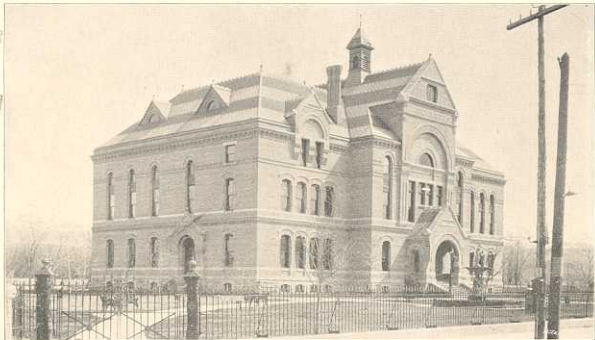
STATE CAPITOL BUILDING.
